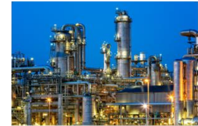
Industrial Control Systems (Mission Secure Inc)
