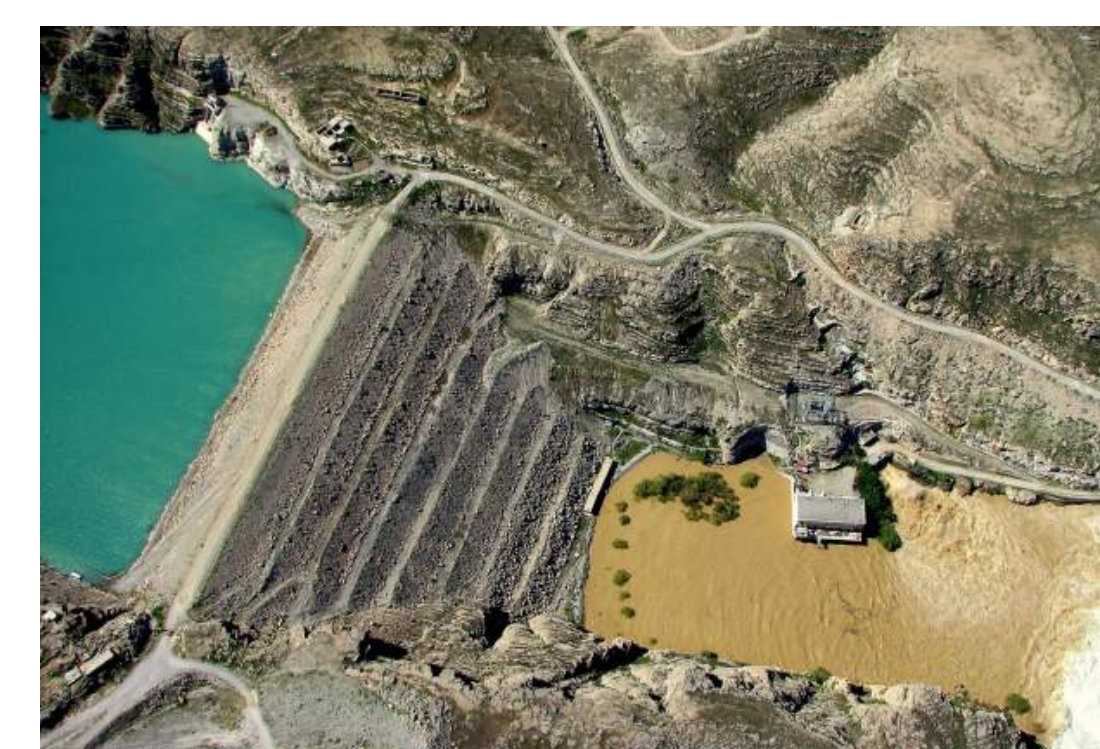
Kajaki Dam, essential for hydropower generation and industrial development
